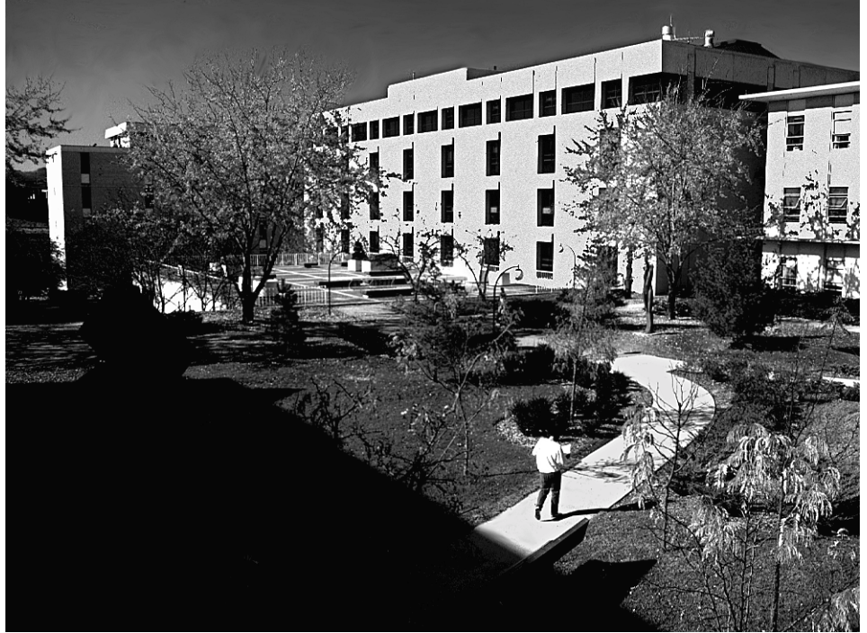
Rigge Science Building viewed from the Southeast.
